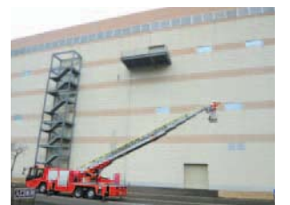
Joint training with the fire station
